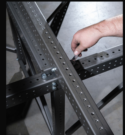
Crossbar being fastened.
